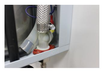
Water piping and evaporation chamber: Scale accumulation can restrict the flow of water. Regular maintenance is required to ensure proper operation of the humidifier.
